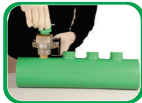
HEAT UP THE WELD-IN SADDLE AND ID OF THE PIPE WITH PROPER DIE'S
